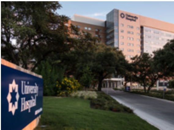
Outside of Building: University Hospital
